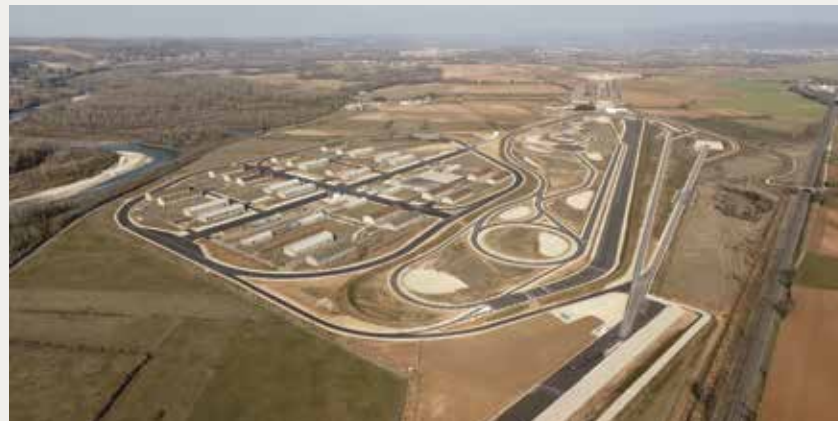
Aerial view of the Transpolis testing platform located in the former Fromentaux military base in Saint-Maurice-de-Rémens
