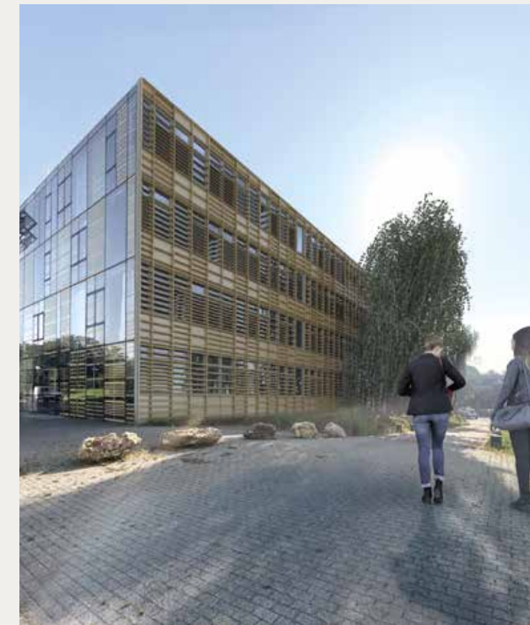
Renovation of the south façade of the Lavoisier building in Champs-sur-Marne
